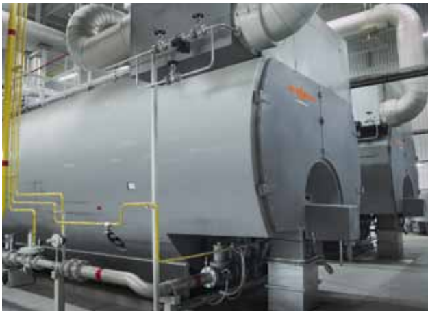
Steam boiler with superheater at Klaipėdos Kartonas, Lithuania
