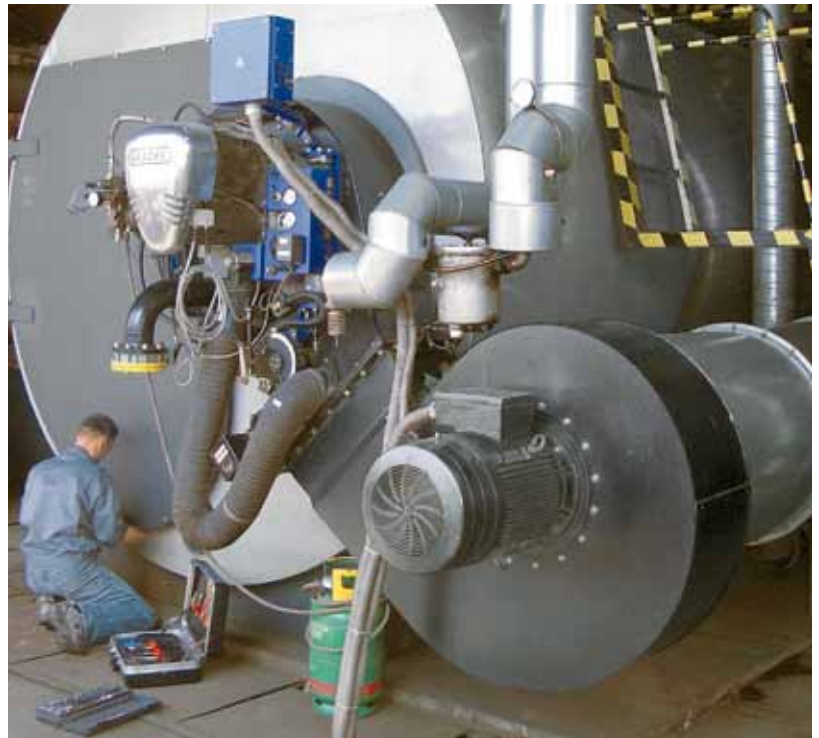
Boiler undergoing maintenance
