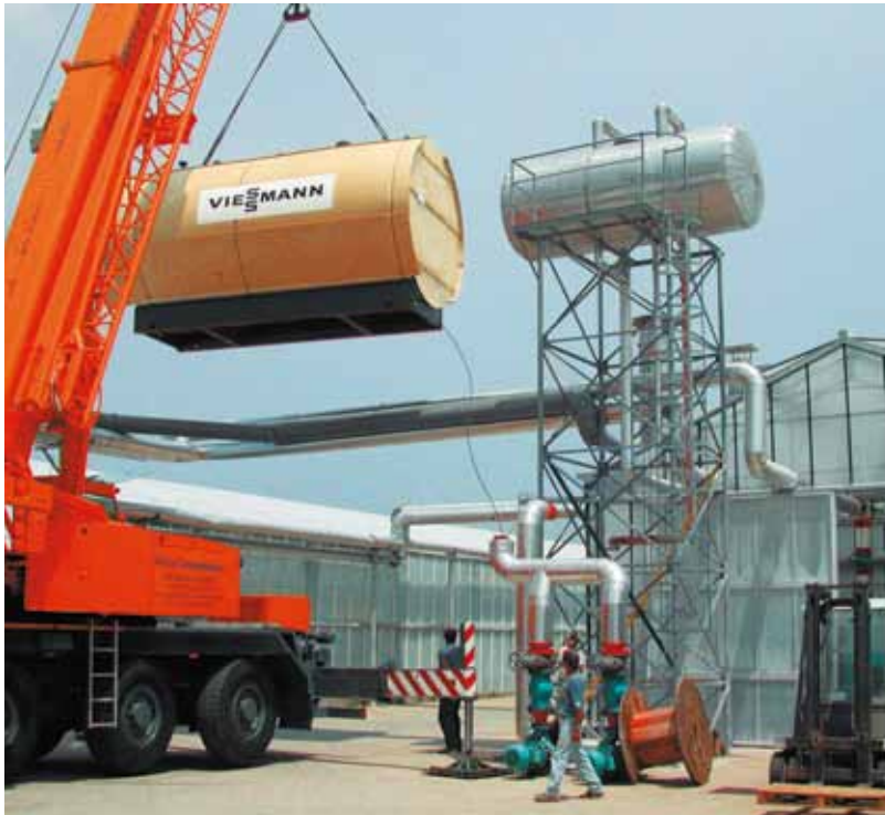
Installing the Vitomax by mobile crane
