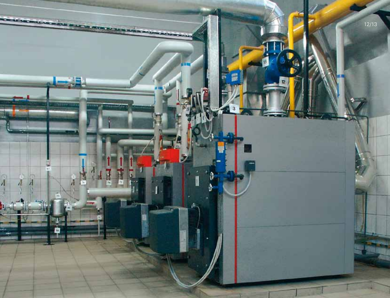
System with one Vitoplex 100-LS low pressure steam boiler and two Vitoplex hot water boilers
