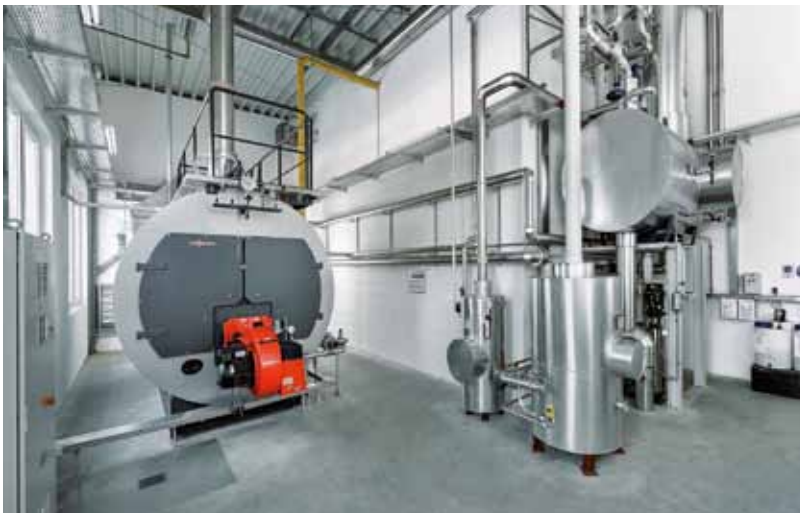
Vitomax 200-HS, 4 t/h, 16 bar, StoVerotec, Germany
