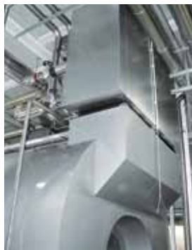
Economiser fitted on a Vitomax 200-HS
