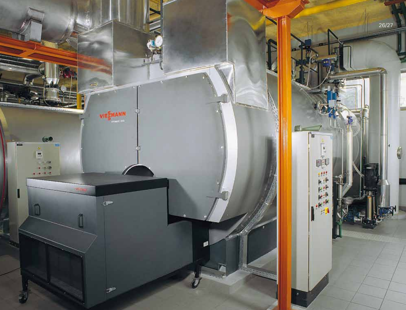
Vitomax 200-RS steam boiler with waste heat utilisation at the Maribor hospital, Slovenia (6 t/h, 13 bar saturated steam)
