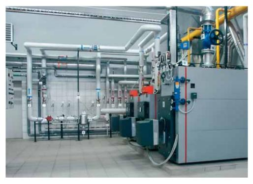
Typical application for smaller industrial premises: a Vitoplex LS (front) and two Vitocrossal boilers are in use here
