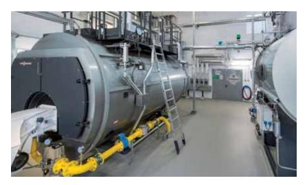
Vitomax HS with a steam output of 6 t/h and 10 bar
