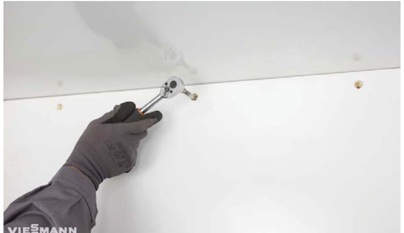
Cold room assembly
